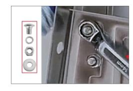
4 Connect the cross bars (C) to the triangle side panels (B) and fix it by the bracket attachment bolt kits (D). Adjust the rubber vibration absorbing pads (G) and place your heat pump. Then put the nuts of condenser attachment bolt kits (F) on it, install the screws of condenser attachment bolt kits (F) to settle the heat pump.
