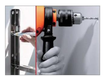
③ Insert the concrete expansion bolts (C) and mount the L-shaped foldable brackets (A) on the wall.
