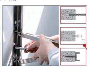
4 Adjust and put the rubber vibration absorbing pads (E) on the foldable brackets (A), then place your heat pump on it. Put the nuts of the condenser attachment bolt kits (D) on the foldable brackets (A), install and tighten the screws of the condenser attachment bolt kits (D) to settle the heat pump.
