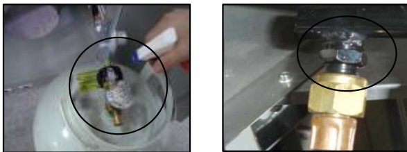
Gas Connection Leak Check
