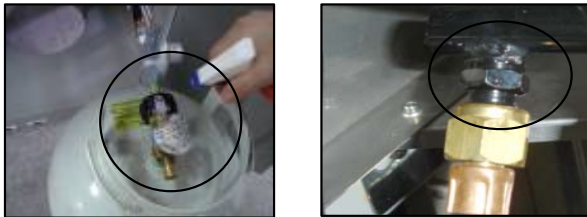
Gas Connection Leak Check
