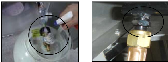
Gas Connection Leak Check
