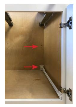
In a standard Base Cabinet there are two locations a Roll-out Tray can be installed, indicated by the two sets of pre-drilled holes on the back panel.
