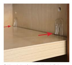
Cabinet shelves feature locking shelf pins. To release, simply push in the tab and lift the shelf
