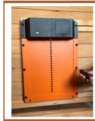
**4** Screw in the door gently. **Do not over-tighten the screws, or the door will not move.**
