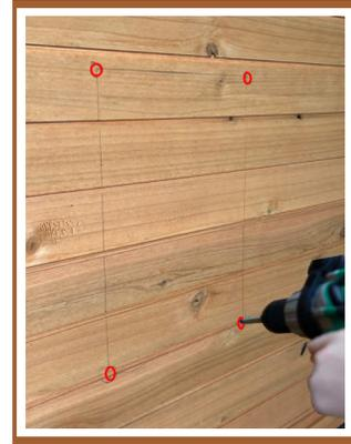
**2** Drill in the corners before sawing the opening area off.
