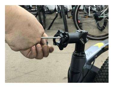
2. Attach the handlebars as shown below by first removing the locking plate's Allen screws.
