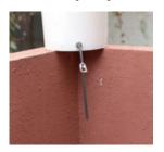
Connect filter according to arrow in the direction of water flow.
