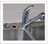
**Fixing to the Sink.** Try to install the faucet on the sink surround if possible, using one of the mounting holes already available, remove the cover, make sure you have clear access above and below.
