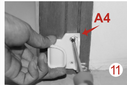
Fix A4 with screws on the surface firmly.
