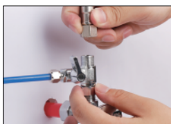
Connect the flexible hose
